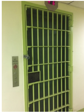
Elevator shaft in the Centre Street DOP adult operations office.
