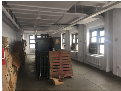
Renovation in progress, 2018.
